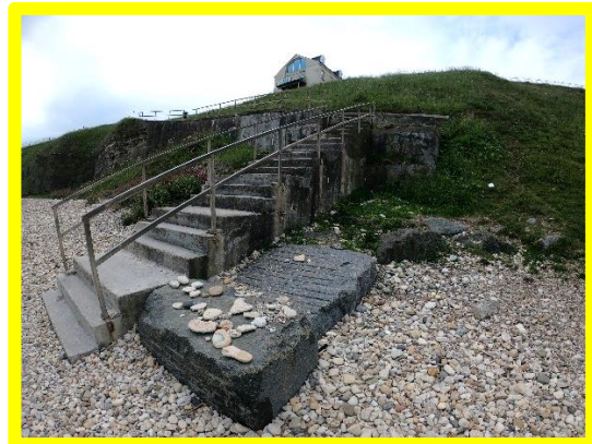
Access ramp and steps (/0103C07)
