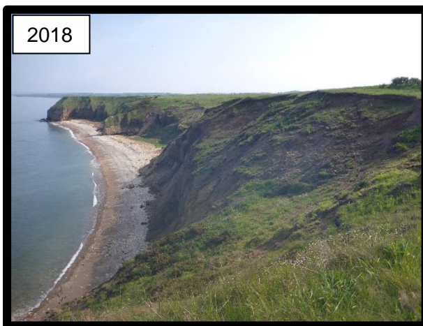
Unnamed Bay fronting Easington Colliery - 2018 (/0201C01)
