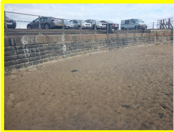
Vertical rear wall recently repointed (circa pre 2018) (/0104C05)
