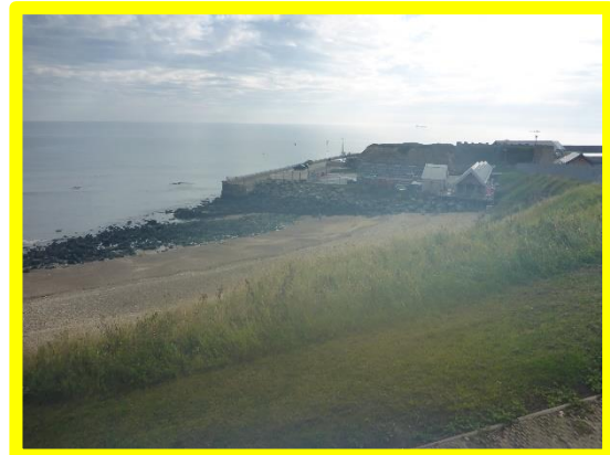
Revetment preventing outflanking of the North Pier(/0104C02)
