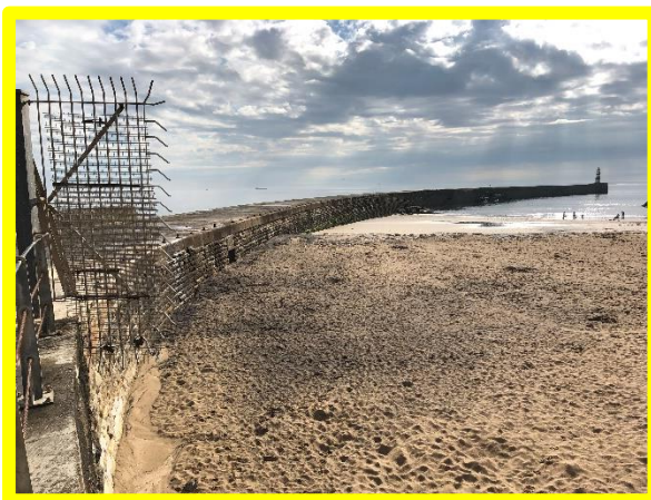
Seaham Harbour North Pier Inner Face (0104C03)
