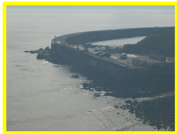
Seaham Harbour North Pier Outer Face (0104C03)
