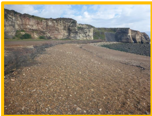
Eroding colliery spoil on Blast Beach (/0103C07)
