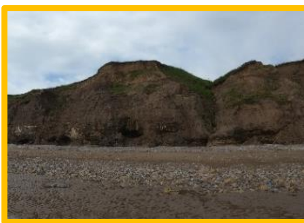
Glacial Till slumping along the majority of the frontage (/0804C01)
