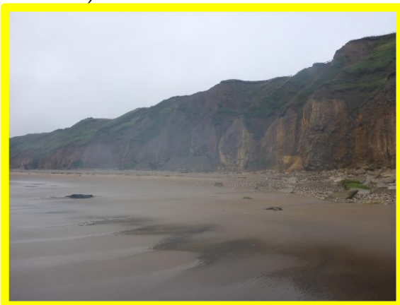
Large-scale slump of softer material (/0301C01)
