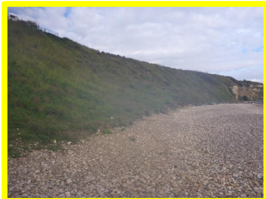
Local slumps in cliffs (/0103C06)
