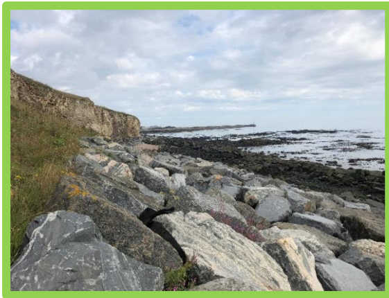
Rock revetment from South Pier to Chemical Beach (/0105C01)
