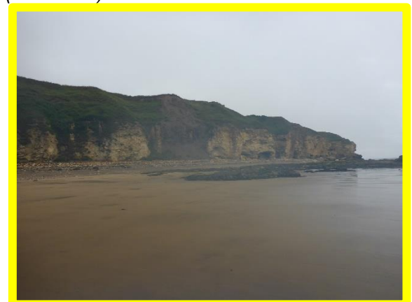
Large-scale slump of softer material (/0301C01)
