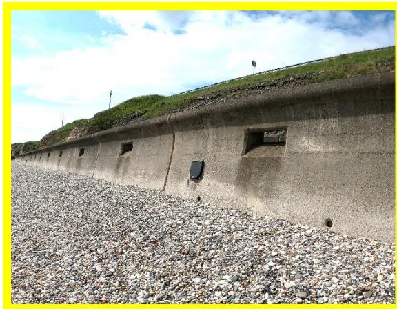
Seaham sea wall (/0102C01)
