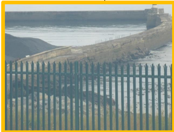
Seaham Harbour South Pier (/0104C17)
