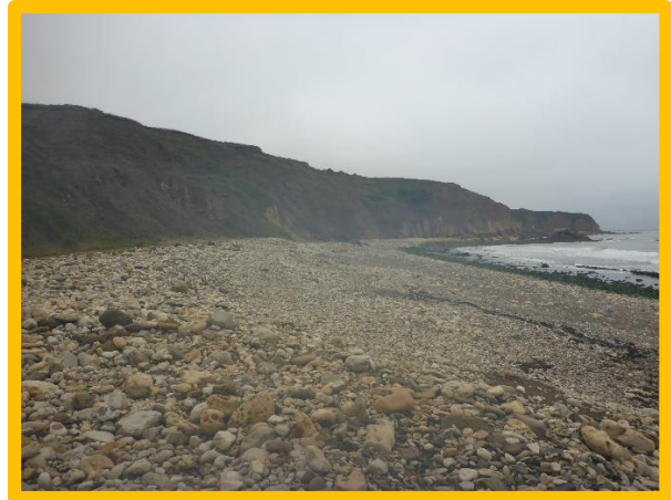
Actively eroding section of cliff in between shot Rock and Loom. (/C0201C01)
