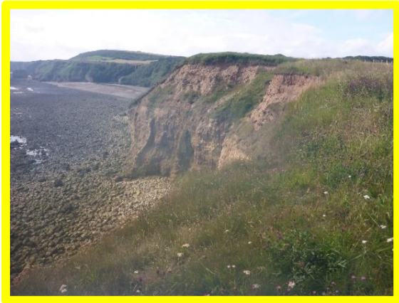
South side of Chourdon Point (/0201C01)
