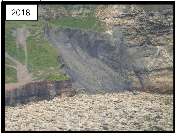
Erosion of informal beach access - 2018 (/0103C07)
