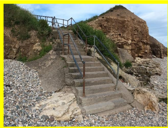
Access steps adjacent stone revetment (/0804C01)
