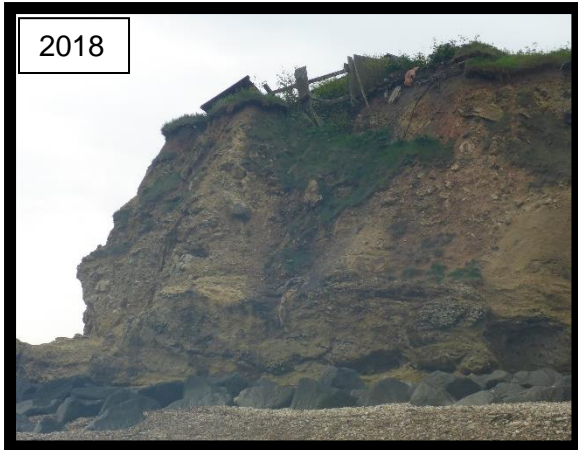
Erosion affecting fence line of properties to south Dawdon Dene Outfall -2018 (/0103C02)
