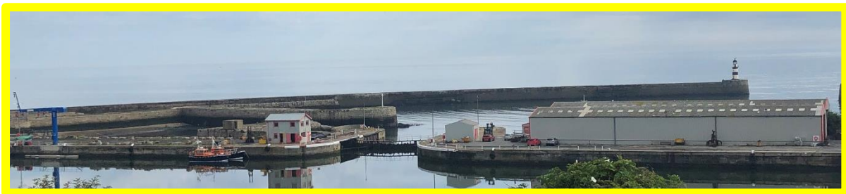
Seaham Harbour North Pier Inner Face (0104C03)
